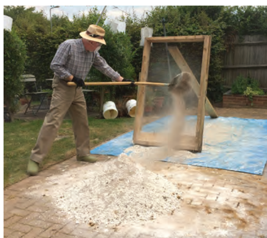
Fig. 11 (Above) When the lime has finished slaking, it is turned with the shovel to mix it with the dry sand; this starts to break down some of the lumps of lime and aggregate.
