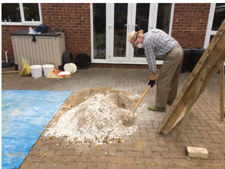
Fig. 11 (Above) When the lime has finished slaking, it is turned with the shovel to mix it with the dry sand; this starts to break down some of the lumps of lime and aggregate.
