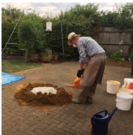
Fig. 7 (Far left) The measure of sand is formed into a ring and the appropriate volume of quicklime is placed in the middle.
