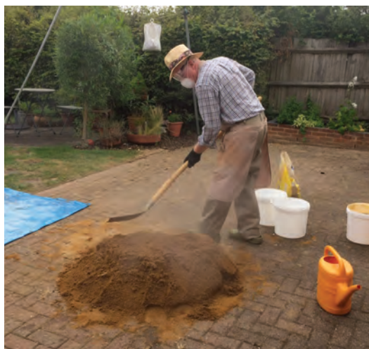
Fig. 9 (Far left) The sand is drawn quickly over the quicklime to cover it fully as slaking starts.
